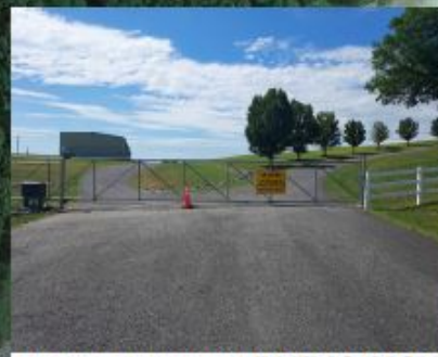
INSTALLED WARNING SIGN
